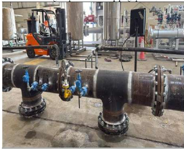
During the pressure test of piping spools
