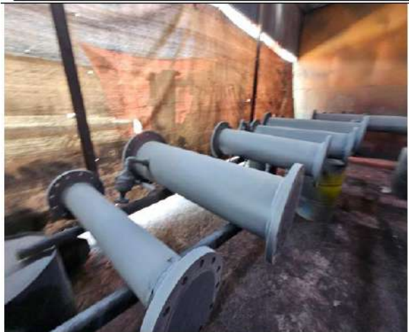
Blasting inspection of piping spools
